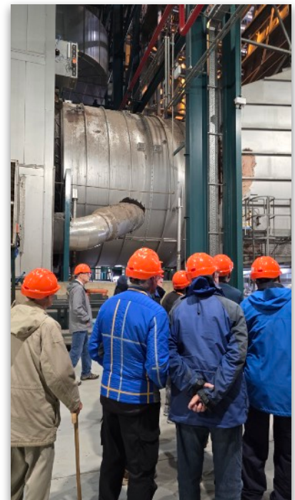
Duct between gas turbine and boiler
