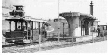
At Black Rock a new station was built to replace the 1937 building which had suffered badly during the war. Most of the steelwork for the platform shelters at 'Half Way' and 'Black Rock' came from wartime defences and aircraft scrap. The 'art-deco' style of station was designed to blend in with the architectural style of the Lido at Black Rock.
