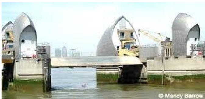
This picture shows the barrier in the maintenance position for cleaning. In this position it is completely out of the water so that all surfaces can be accessed.
