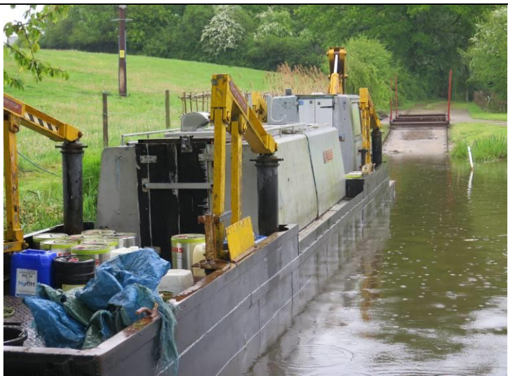
The work boat at the bottom of the slipway where boats are hauled out of the canal for maintenance.
